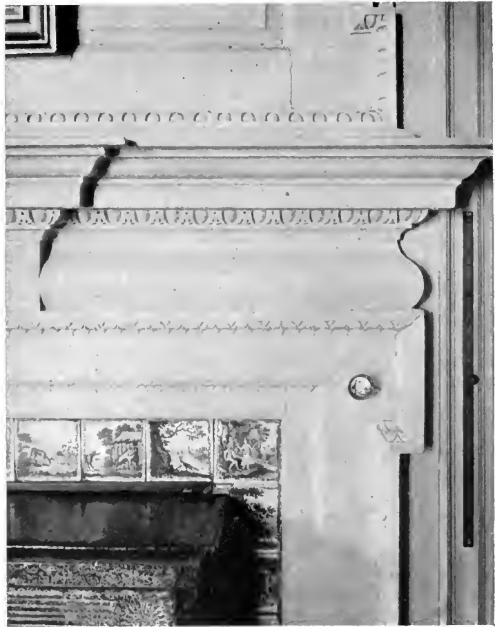
CORNER OF WEST PARLOR MANTEL PIERCE-NICHOLS HOUSE, SALEM, MASS. SAMUEL McINTIRE, ARCHITECT
